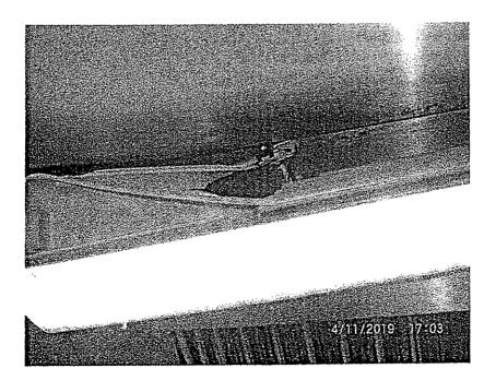
The overhead light fixtures in the main kitchen were in very poor condition and cannot be cleaned and pose a risk of physical contamination of food. Renew or repair the light fixtures and leave in a sound easy to clean condition.
