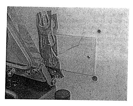
12. The wash hand basin was in poor repair and had a missing bolt. Ensure that this is repaired and maintained as this can also cause physical contamination of foods.
