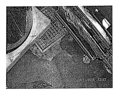
The floor covering throughout the kitchen areas and walk in fridges was in very poor condition. This does not allow adequate cleaning and can also be a trip hazard. Renew or repair the floor covering and leave in a sound easy to clean condition.
