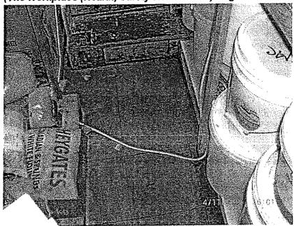
2. During the inspection, I noted that your walk-in freezer had a leak and was causing ice buildup on the floor. This can cause slips to staff due to slippery floor surfaces. Ensure this is defrosted, cleaned and if necessary provide an anti-slip mat.
