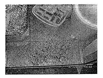
The floor covering in the kitchen was very dirty especially at floor/wall junctions and behind or below equipment. The layout, design, construction and siting and size of the food prmises are to be in such way as to permit adequate maintenance, cleaning and disinfection. It is not an excuse to say that you cannot move the equipment to clean hard to reach surfaces. You must ensure that these areas are thoroughly clean and maintained in a clean condition.
