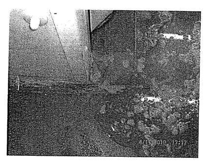
The floor covering throughout the kitchen areas and walk in fridges was in very poor condition. This does not allow adequate cleaning and can also be a trip hazard. Renew or repair the floor covering and leave in a sound easy to clean condition.
